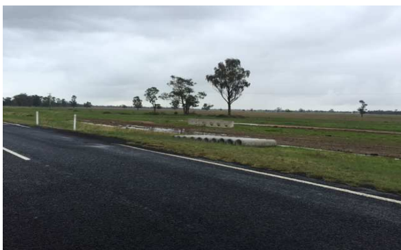
B55 Castlereagh Hwy (SH18) - Culvert works
