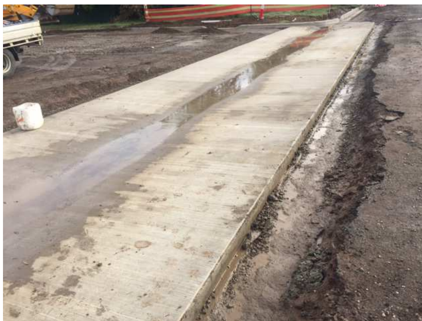
Dubbo Street Coonamble – Dish drain construction
