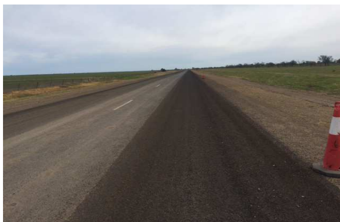
SR2 Tooraweenah Road – Shoulder Widening/Heavy Patching 28 May 2015
