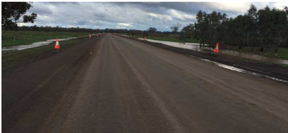
Warren Road MR 7515 Construction
