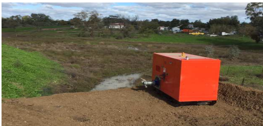
Coonamble Levee Flood Pump Platform
