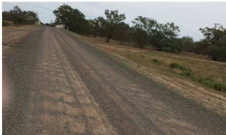
Wingadee Road – east of the bridge
