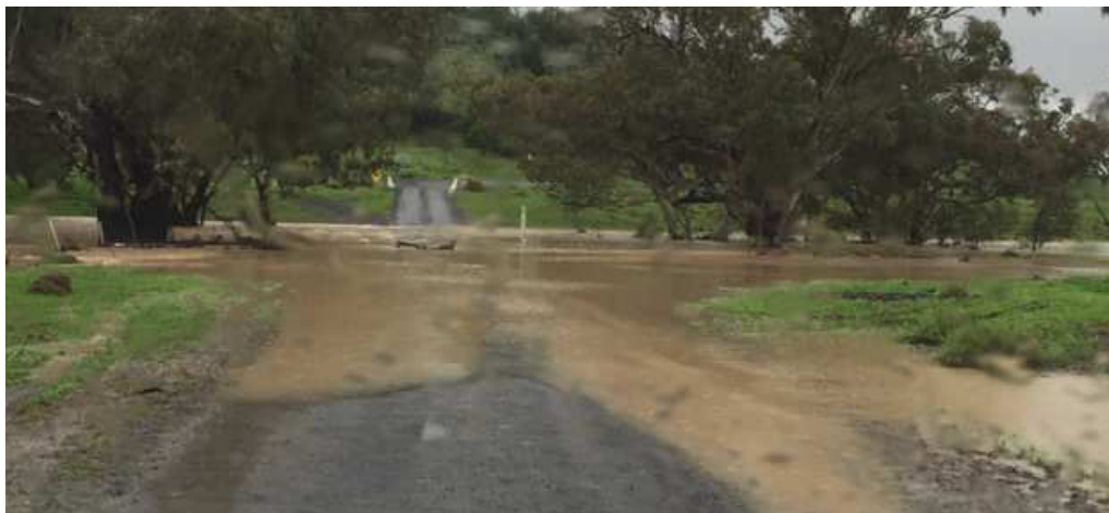
Mt Magometon Quarry access road flooded
