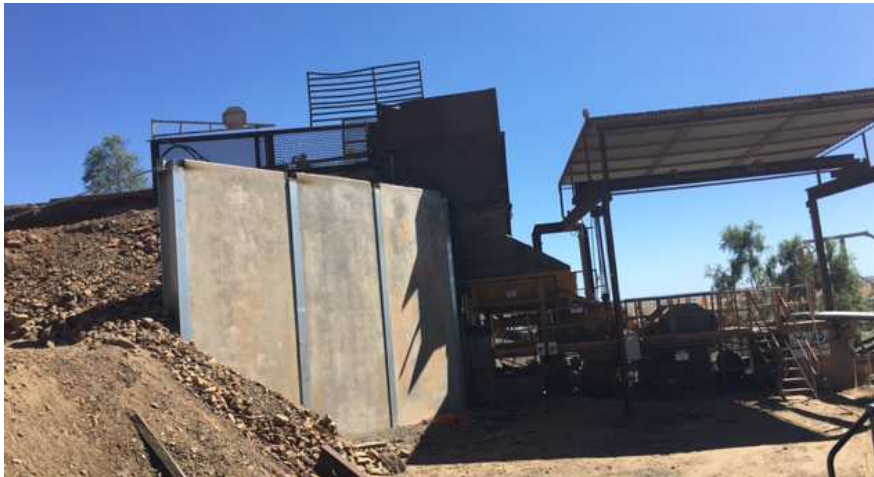
Coonamble Quarry Retaining Wall Construction
