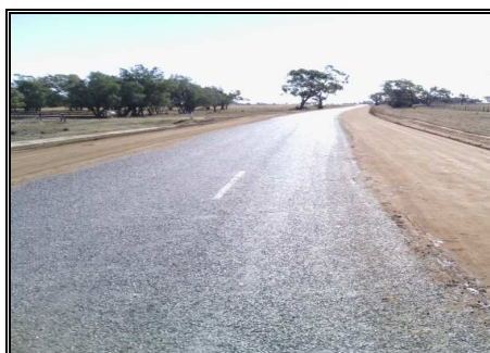
SR86 Shoulder Grade
