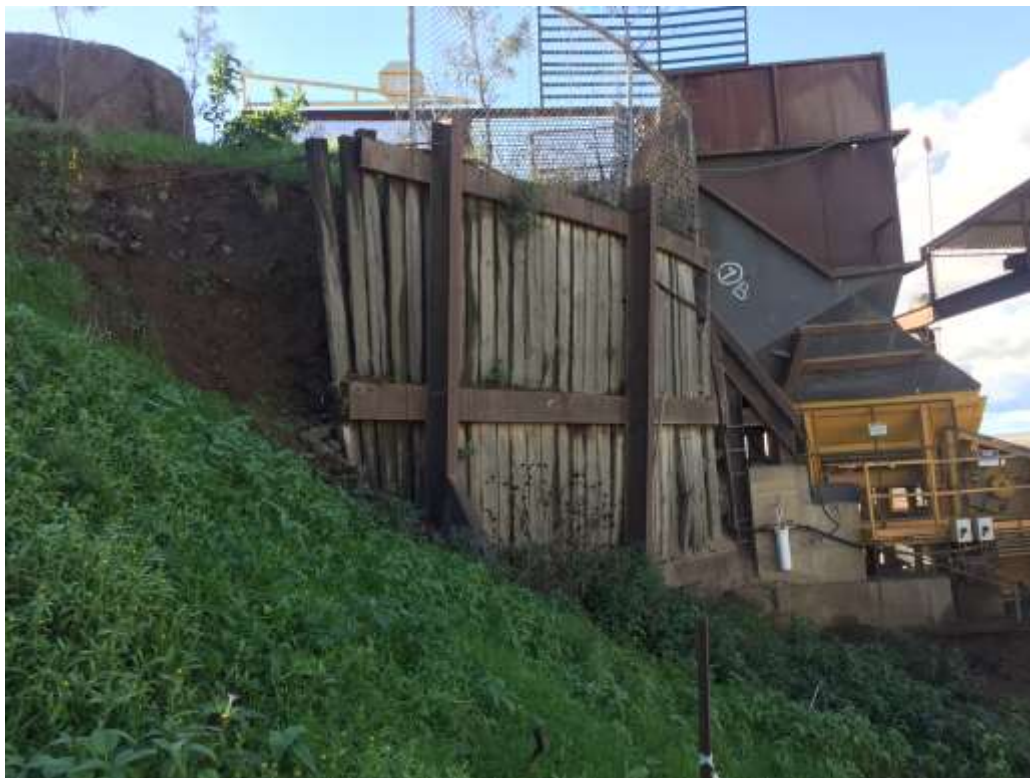
Mount Magnet Quarry – Crushing Plant Retaining Wall
