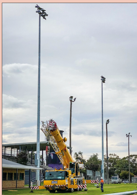
A crane completes the job of lifting new lighting poles into place at Coonamble Sports Ground.
