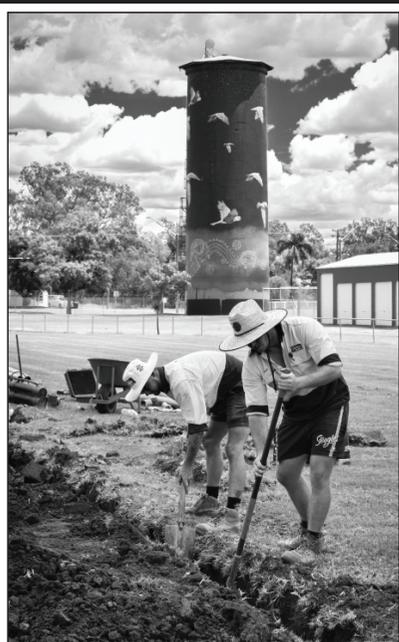
Workers continue trenching for conduit to install new lighting at Coonamble Sports Ground.
