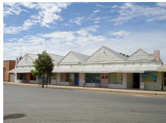
Plate 4.6: Rustic Inter-War commercial buildings.
