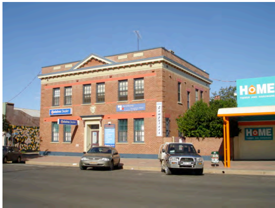
Plate 4.3: The former Bank of NSW.
